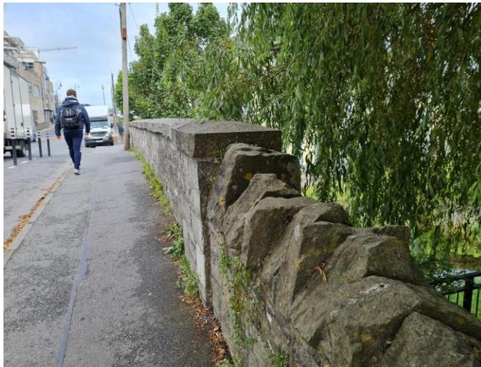
Fig. 56: Stone rubble wall on the approach to William Bridge on the east side of Mill Street
